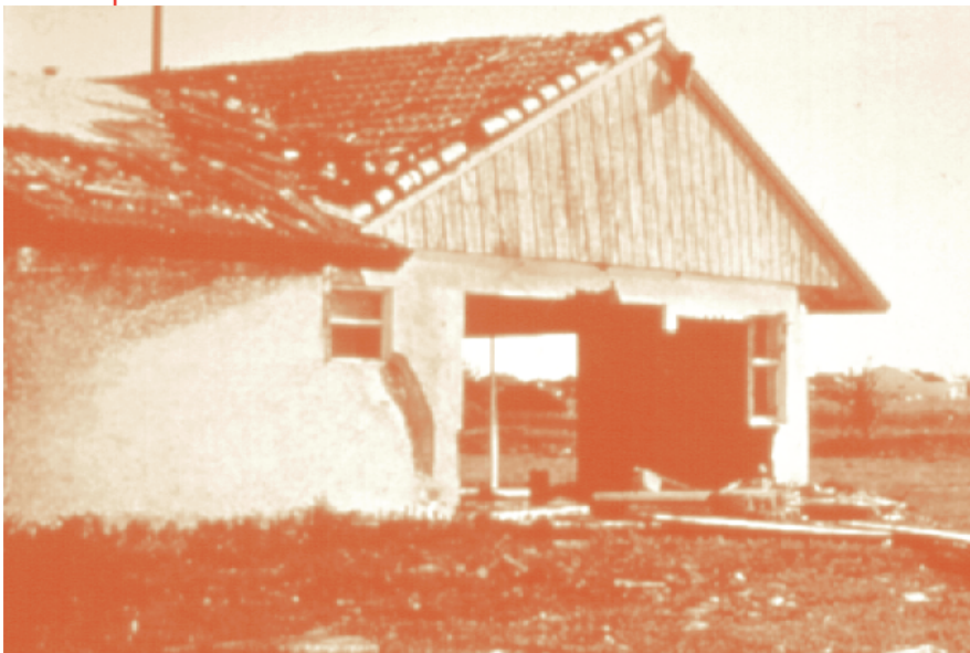
Example of failure of the house envelope.
